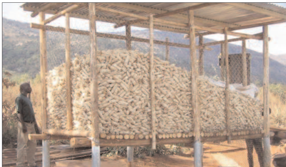
New rodent-proof drying crib for harvested maize built in Swaziland. Strips of metal are placed around each leg, which is too slippery for the rats to climb over. Photo: Steven Belmain
